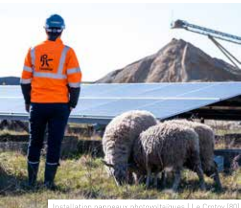
Installation panneaux photovoltaïques | Le Crotoy (80)
